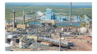
Antelope Valley Station and Great Plains Coal Gasification Beulah, ND. 22,000 gpm water withdrawal in a zone that receives 14 in. of annual rainfall. (EIS-0072-FEIS, 1980) Once through thermoelectric power total water use 2015 (USGS circ. 1441)
