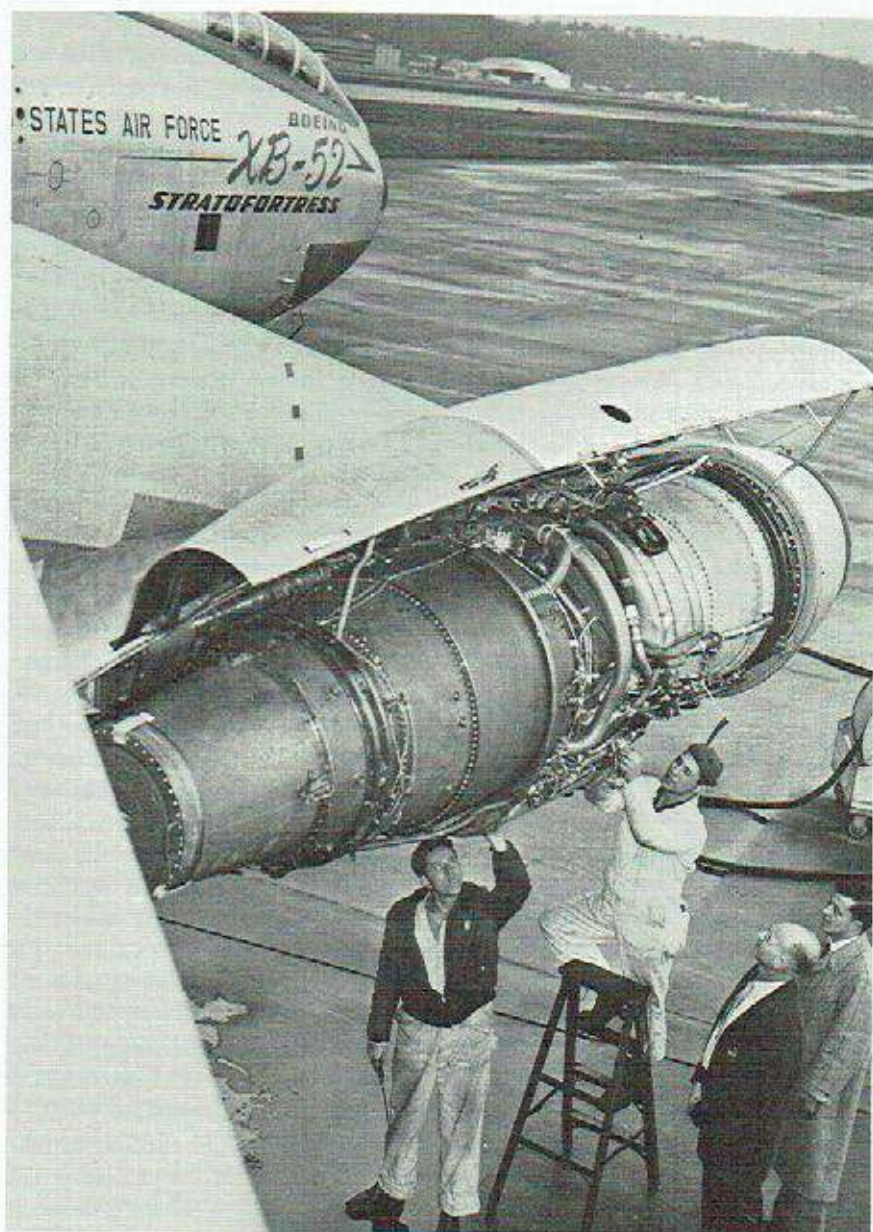
Early JT3, designated J57 by the military services, is shown being installed on experimental Boeing B-52 bomber. The eight-engined B-52 was the first production home for the JT3.
