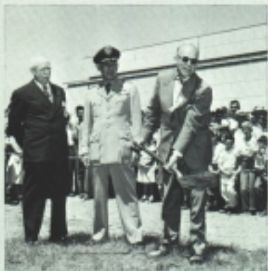
Expansion of the Grafton plant to house the 35,000- and 50,000-ton hydraulic presses took place in 1951, five years after the 18,000-ton press began operation. Above, George Motherwell, vice-president of Wyman-Gordon, breaks ground as George Fuller, former chairman of the Board, and Gen. K. B. Wolf, U. S. Air Force, Wright-Patterson Air Force Base, look on at June 26, 1951 ceremony.
