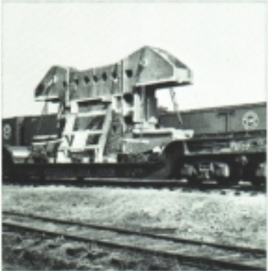
Movement of components was a major undertaking.
